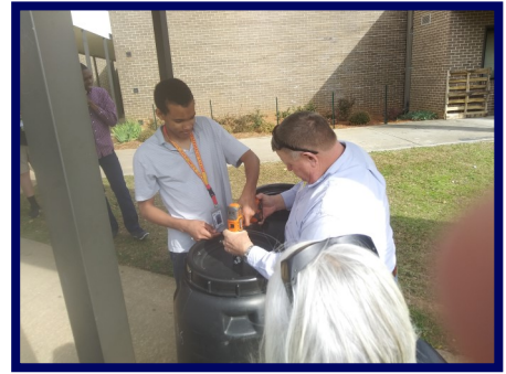
Student tries his hand at drilling inlet holes for rain to enter barrel.
