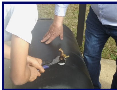
Student positions spigot using adjustable wrench.
