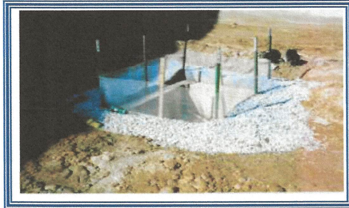
Hardware Fabric and Stone Inlet Protection
