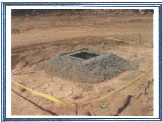
Block and Gravel Inlet Protection
