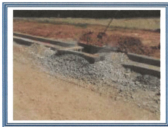
Block and Gravel Inlet Protection
