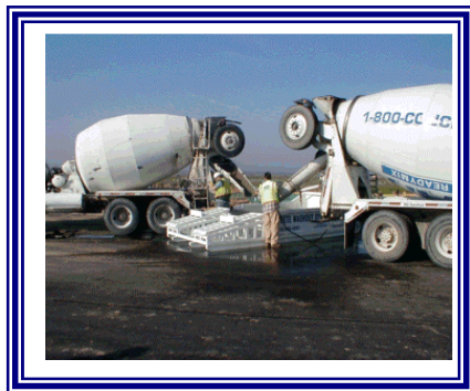
Concrete Truck Washout
