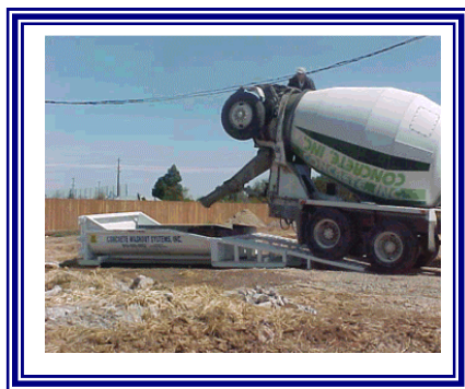
Concrete Truck Washout
